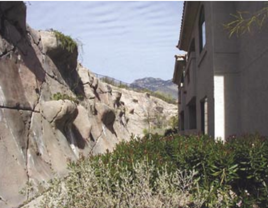
Apartment complex, Tucson, Arizona
