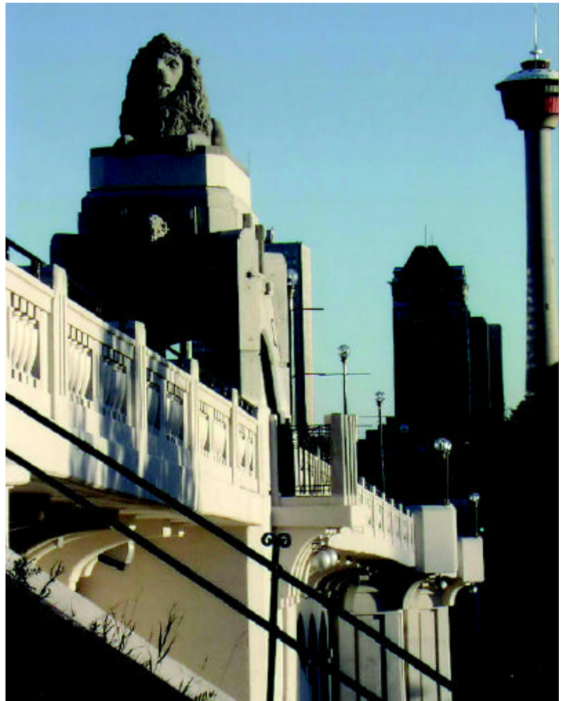
Figure 4: Lion mounted on kiosk on Centre Street Bridge in Calgary.
