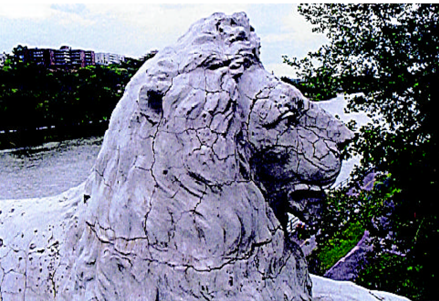
Figure 1: Deteriorated condition of one of the original lions.
