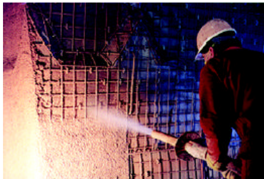
Figure 3: Shotcreting on this project required painstaking care.
