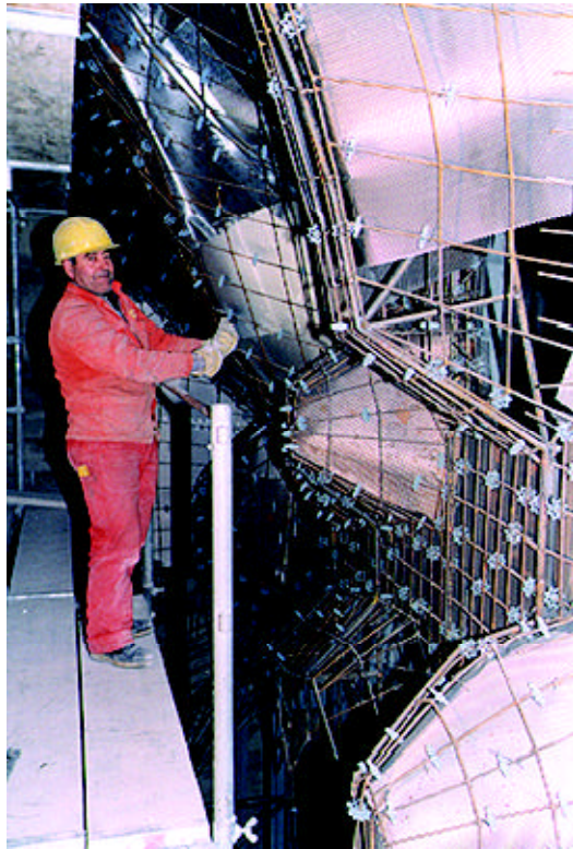
Figure 2: Skeleton with expanded metal fastened behind as “lost formwork.”
