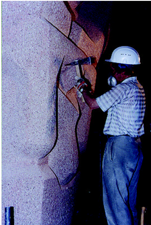
Figure 5: Sculpting of the shotcrete.
