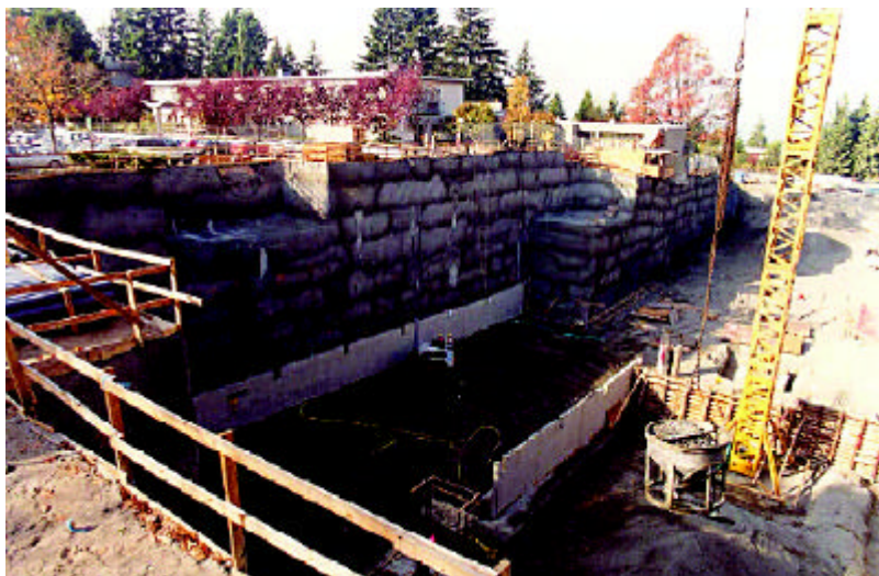
Figure 2: View of finished top-down construction stressed tie-back shotcrete supported excavation.
