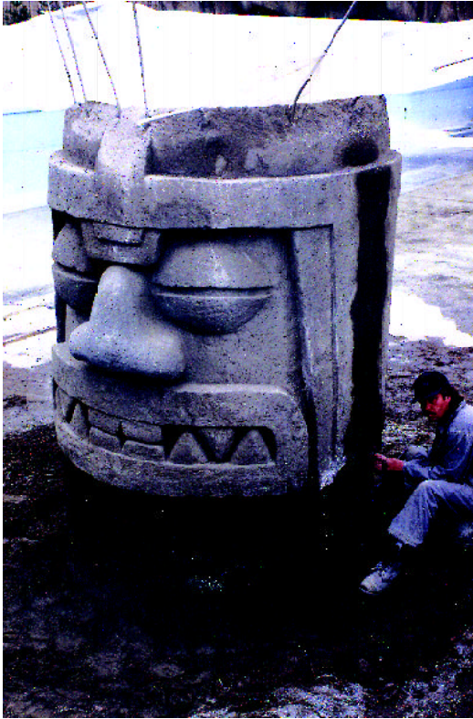
Figure 8: Carving of shotcrete requires artistic skills.
