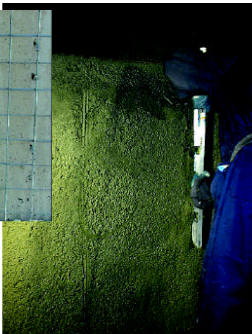
Figure 4: Vertical leveling operation and the groove (bottom).
