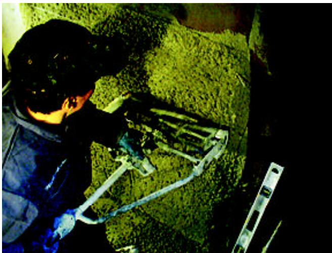
Figure 6: Use of mechanical screeder to do the cutting and the screeding.
