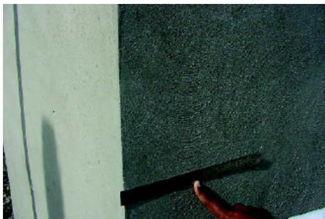
Figure 1: Typical mechanical shotcrete finish.
