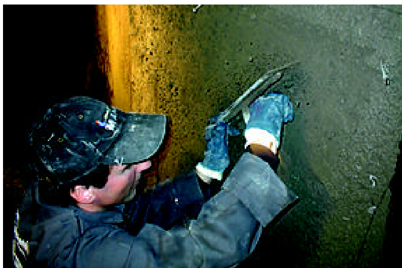
Figure 5: Scratching with the edge of the trowel perpendicular to the surface.
