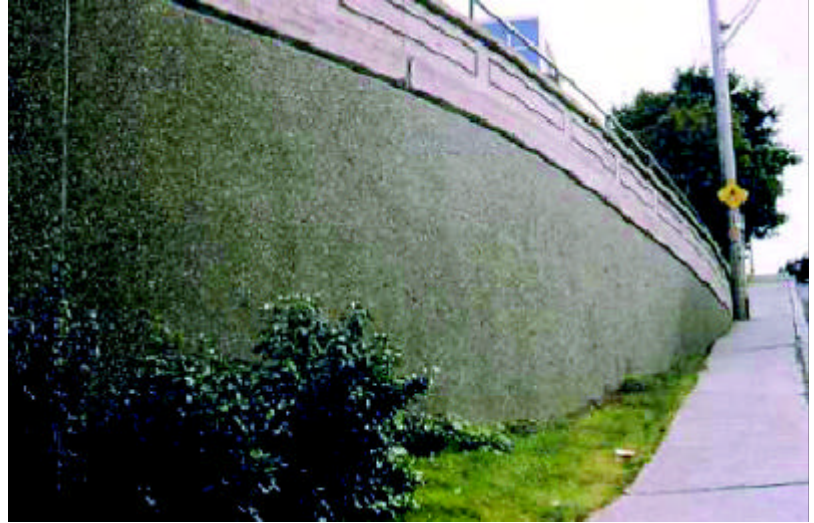
Figure 9: Exposed aggregate shotcrete wall repair in Quebec City.
