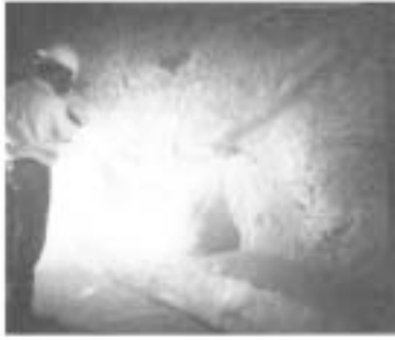
Fig. 17: Bench gunning or 45 deg angle nozzle technique.
