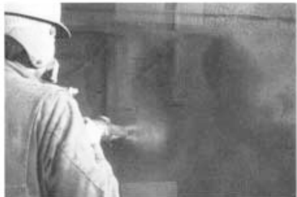
Figure 16: Right angle nozzle technique.
