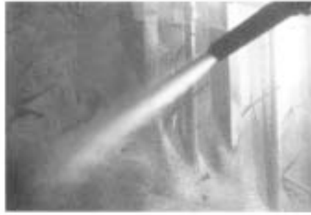
Fig. 17: Bench gunning or 45 deg angle nozzle technique.
