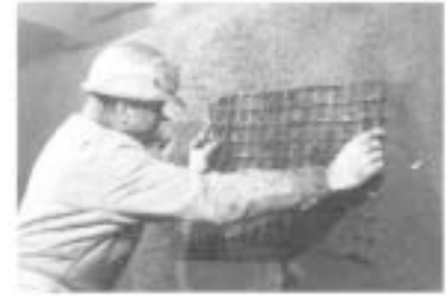
Fig. 18: Removing high spots after gunning.
