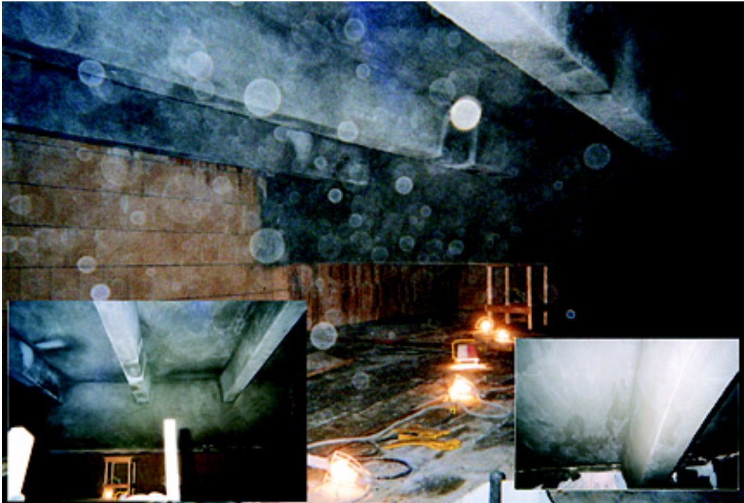
Figure 3: View of the finished surface.
