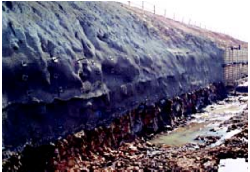
Figure 4: Wet-mix shotcrete soil nails—South Carolina (Photo courtesy of Schnabel).
