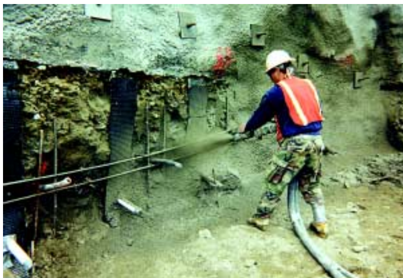
Figure 3: Wet-mix steel fiber-reinforced shotcrete applied for soil nailing—Connecticut (Photo courtesy of Schnabel).
