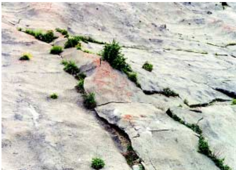
Figure 1: Mesh reinforced shotcrete—frost heave damage—Montana, 1999.
