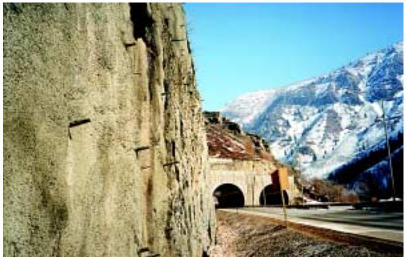
Figure 5: Steel fiber-reinforced shotcrete—Provo Canyon, Utah 1998 (Photo taken 2002).
