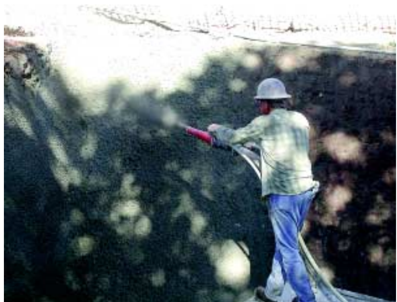
Hand-held nozzling. As height was needed, the nozzleman was raised in a "bucket".
