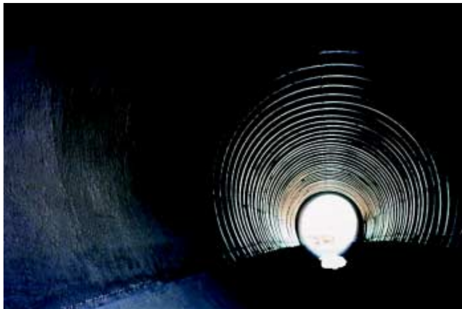
Finished sewer line.
