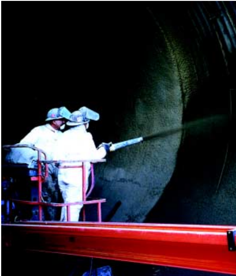
Coastal Gunitite employees shoot the final coating on the walls of the Highland Creek project.
