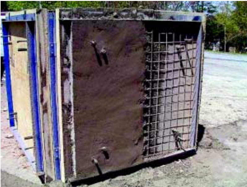
Figure 3: Mesh reinforced South African panel (jointed) after shooting.
