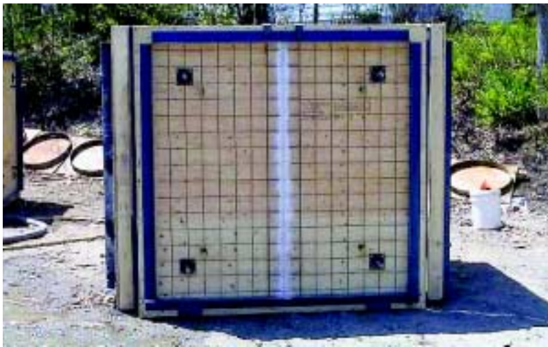
Figure 2: Mesh reinforced South African panel (jointed) before shooting.
