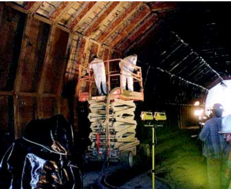
Figure 1: Shotcreting for rehabilitation of highway tunnel.
