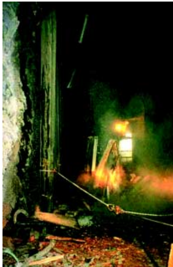
Figure 6: Timber set removal in railroad tunnel.
