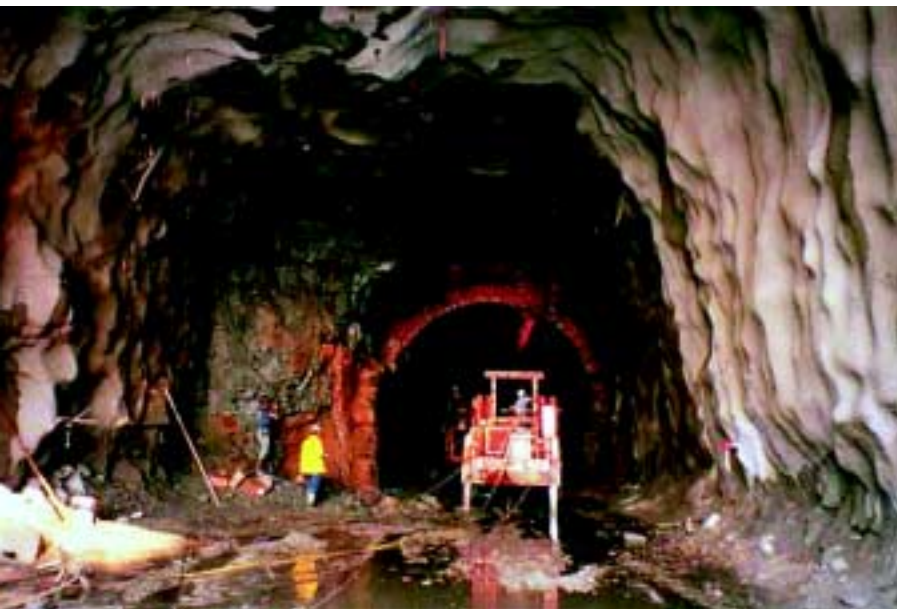
Figure 5: Railroad tunnel clearance excavation: single to double track.
