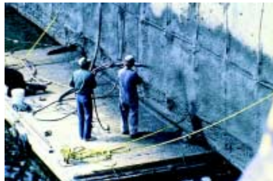
Figure 6: View of shotcrete being applied to berth face from floating barge.
