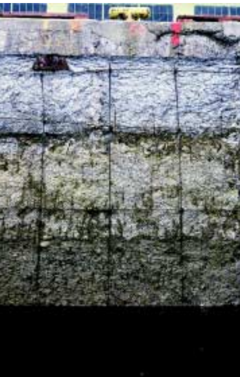
Figure 4: Prepared berth face, with anchor system installed, ready for shotcreting.
