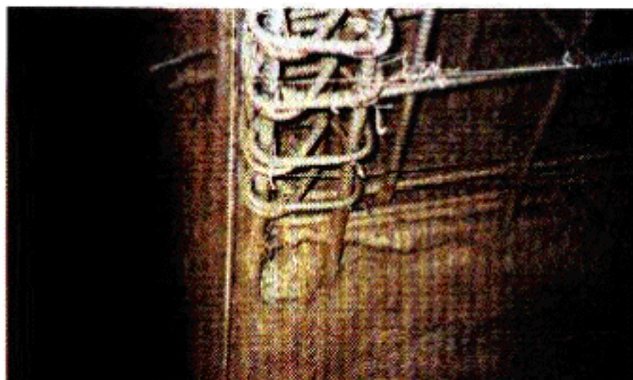
Figure 2: Ground wire delineates finish of a corner without restriction of nozzle trajectory.
