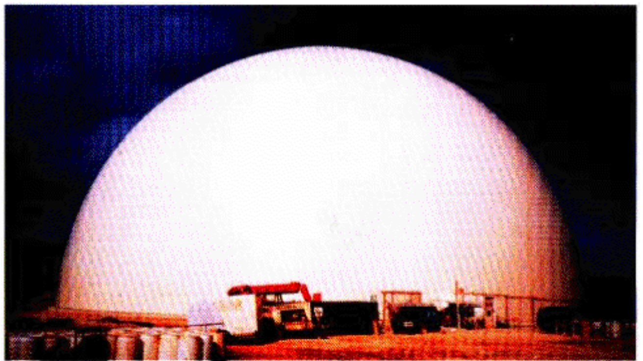
Figure 3: Holnam cement storage dome, Holly Hill, SC.
