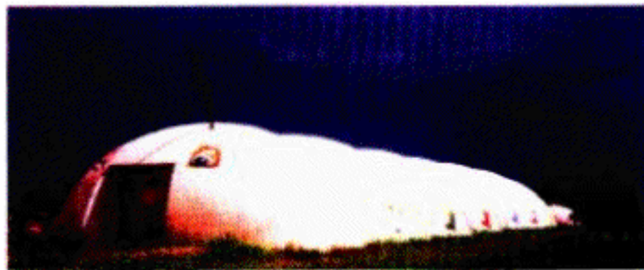
Figure 4. Bruco — the Italian name for caterpillar — houses the Airform manufacturing plant of Monolithic Constructors, Inc. in Italy, Texas. It was built using a single Airform that was shaped as seven interconnected domes. When the Airform was inflated, this shape was automatically achieved.
