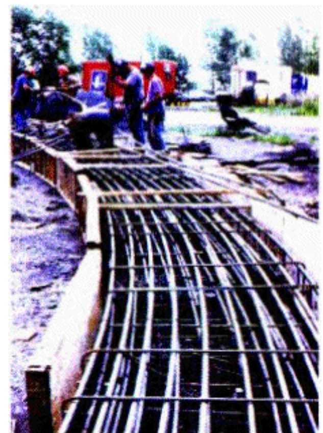
Figure 2: Preparation of ring beam.
