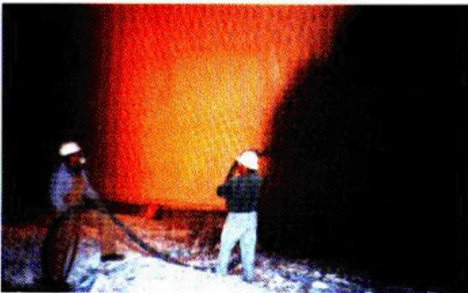
Figure 5: Shooting the first layer over the form.
