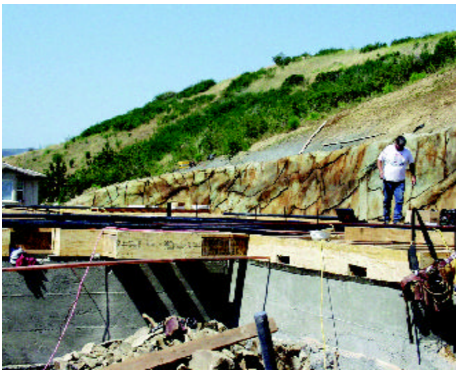
Figure 4: Artificial rock retaining system
