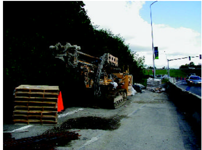
Figure 1: Klemm KR803D drill rig
