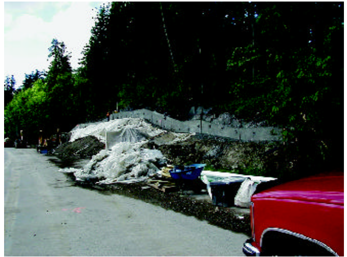
Figure 3: First lift (note elevation changes)
