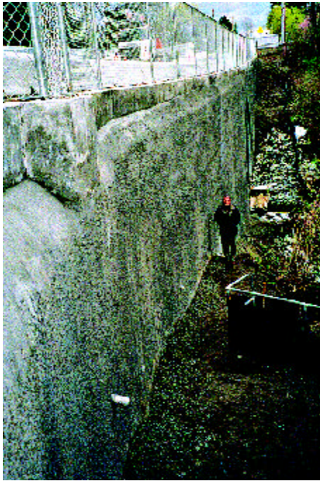
Figure 4. North face after application of shotcrete lining.
