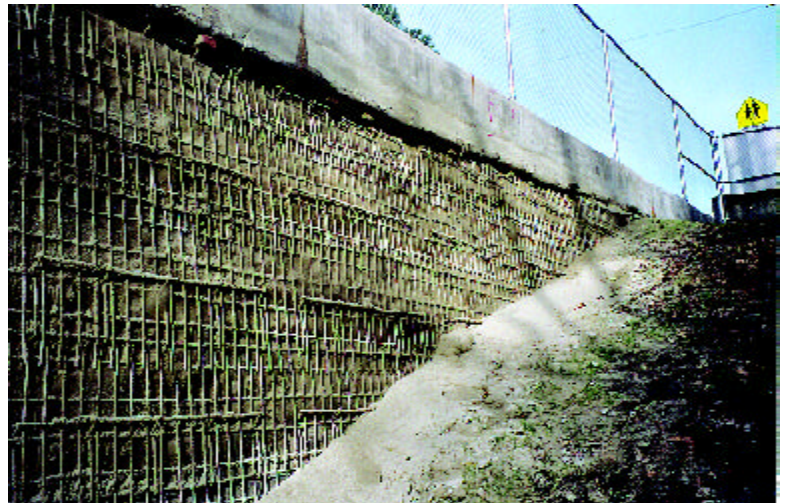
Figure 2. Section of north face after filling voids with sand.
