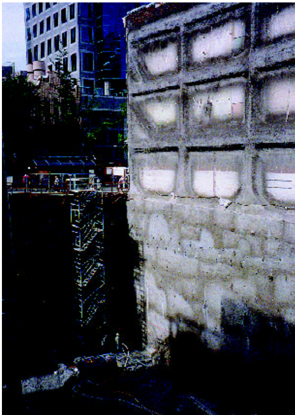
Figure 7: Completed underpinned and shored shotcrete.
