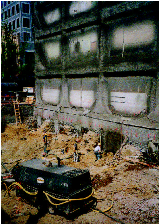
Figure 6: Panel sequence of underpinning.
