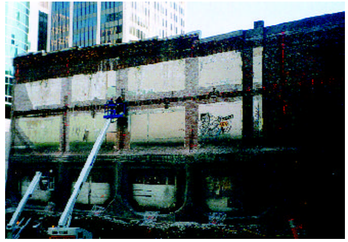
Figure 4: First lift in place and prepping for second lift.
