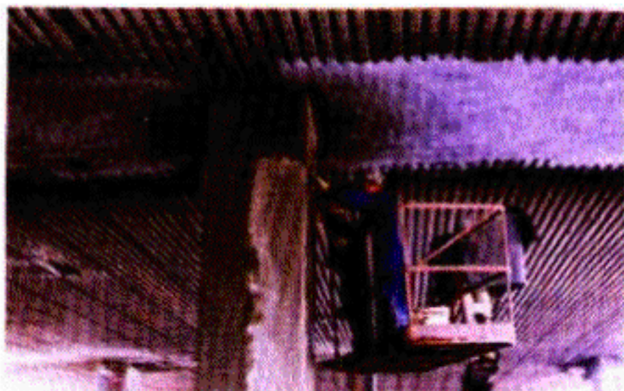
Figure 2. Finishing operation on column after shotcrete application.
