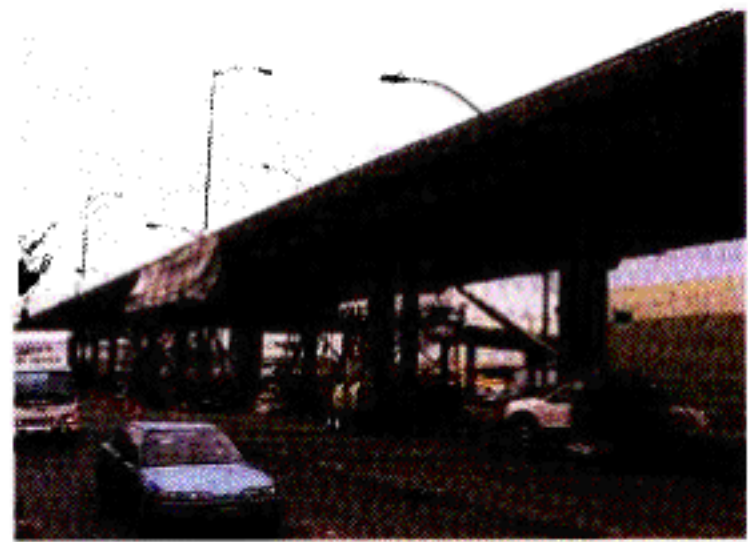
Shooting in progress on south side of bridge.
