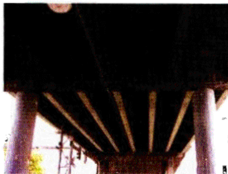
Underside of bridge, prior to shooting.
