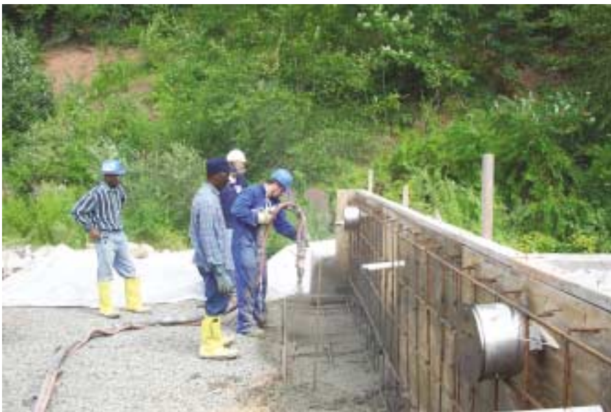
Photo 3: Professor Denis Beaupré instructs three Rizzo employees shooting simulated pool floor and wall, the proper procedure for shooting floor.
