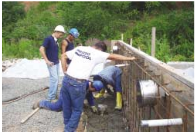
Photo 1: Setting main drain in a fictitious pool wall. Rizzo personnel showing Denis Beaupré (in blue hardhat, kneeling) how to set main drain.
