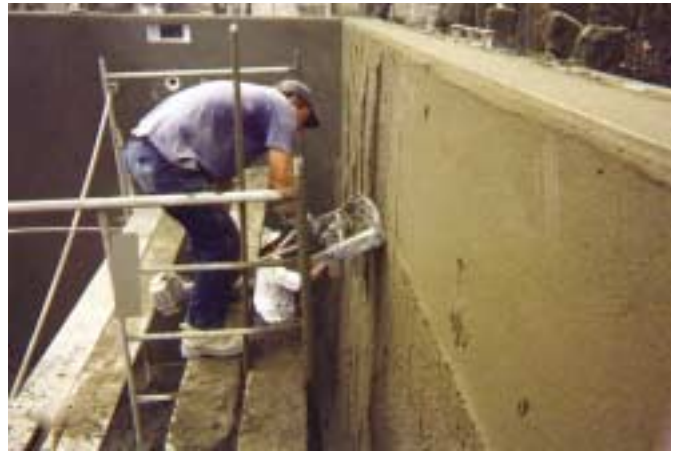
Figure 3: Close-up of the screeding device. Note the wall in the background, made of one monolithic layer of shotcrete and fully finished (no plastering needed).
