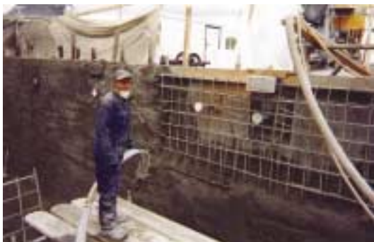
Figure 1: Example of steel layout for a pool being constructed in the city of Quebec. Note the two layers of #10M steel (between US#3 and US#4) spaced at 8 in. (200 mm) in both directions.
