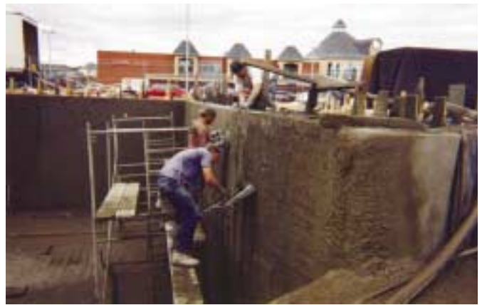
Figure 2: Use of mechanical screed and finishing machine. It took a crew of three craftsmen about an hour to finish the wall.
