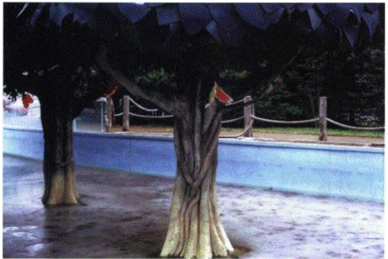
Final shape and texture of shotcrete trees
