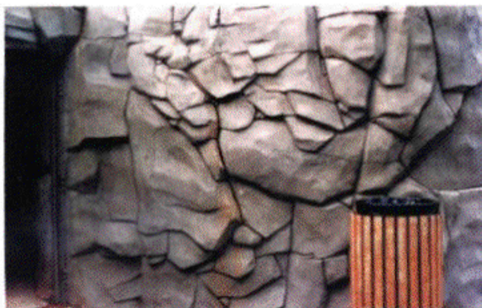
Texturing makes it difficult to tell artificial rocks from the real thing.
