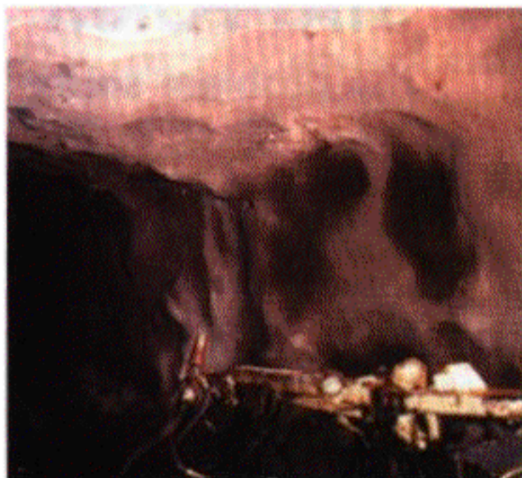
Figure 1. Fiber-reinforced shotcreted heading in a state-of-the-art underground mine.
