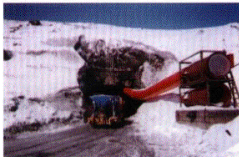
Figure 6: Shotcrete carrier using surface ramp access.
