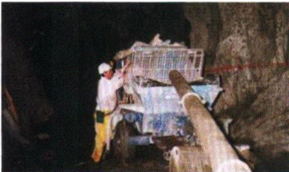
Figure 3. Pump Receiving hopper and delivery pipe.
