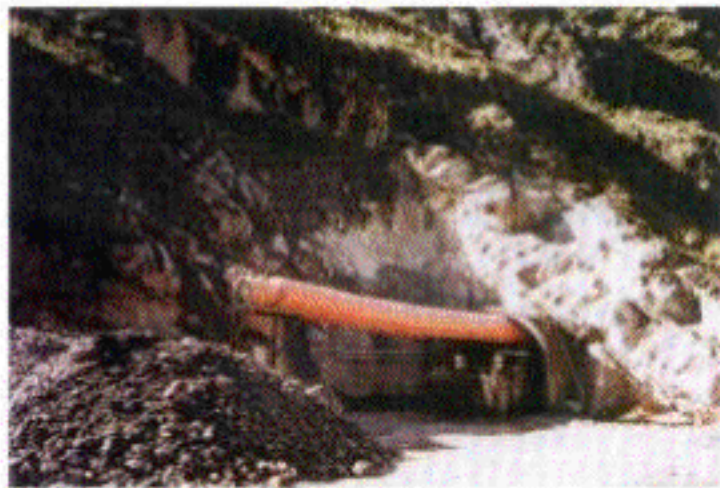
Figure 2. Shotcreted outlet portal, Antamina Decant tunnel in Peru.
