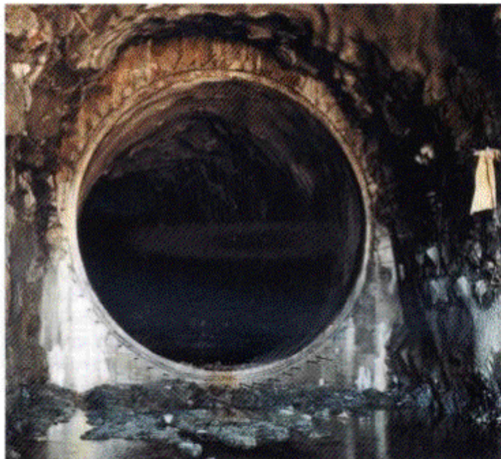
Photo 3. Transition from shotcrete lined tunnel to circular steel lining.
