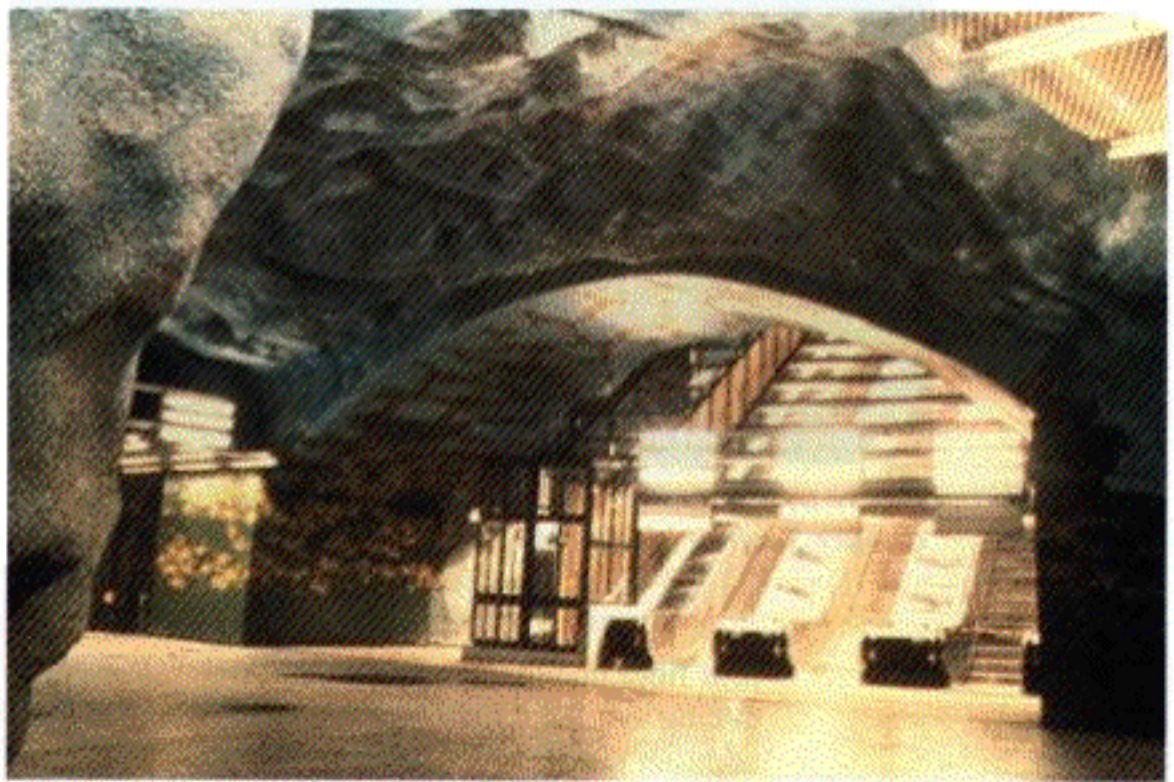
Figure 4. SFRS final tunnel lining of underground metro (passenger railway station) in Stockholm, Sweden.
