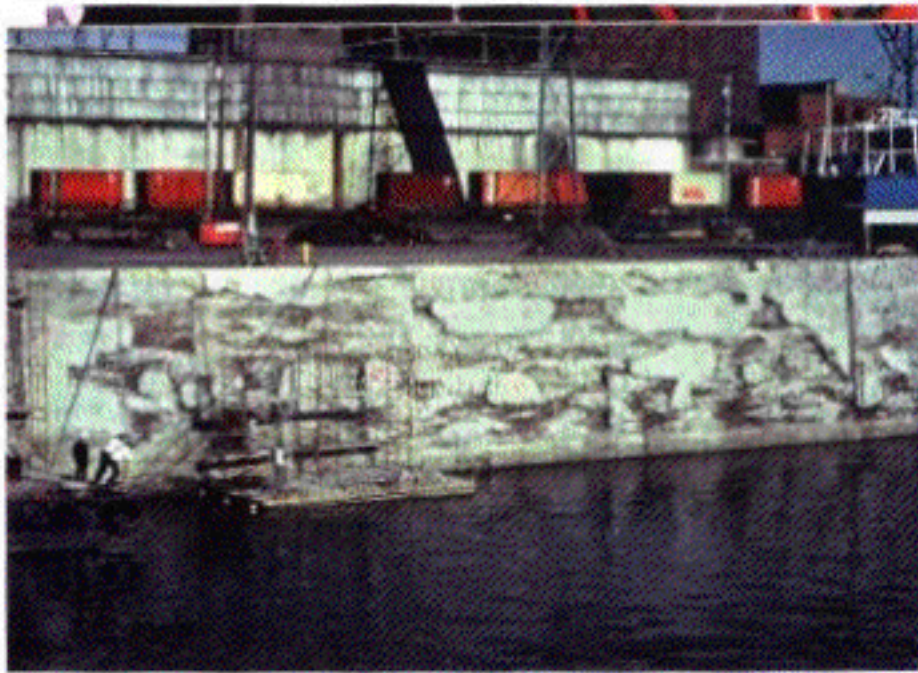
Figure 5: Preparation of shipping berth faces at Port of
