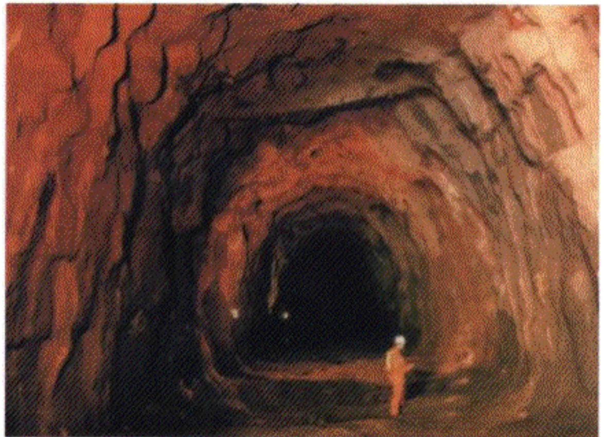
Figure 3. SFRS final tunnel lining, Stave Falls Hydro Electric Project, British Columbia, 1998.
