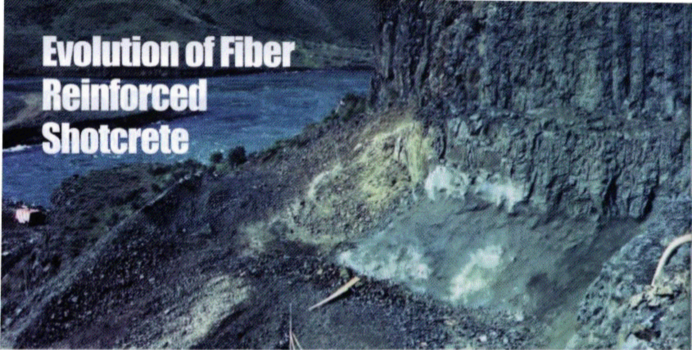
Figure 1. Rock slope stabilization with SFRS, Snake River, Idaho, 1972.
