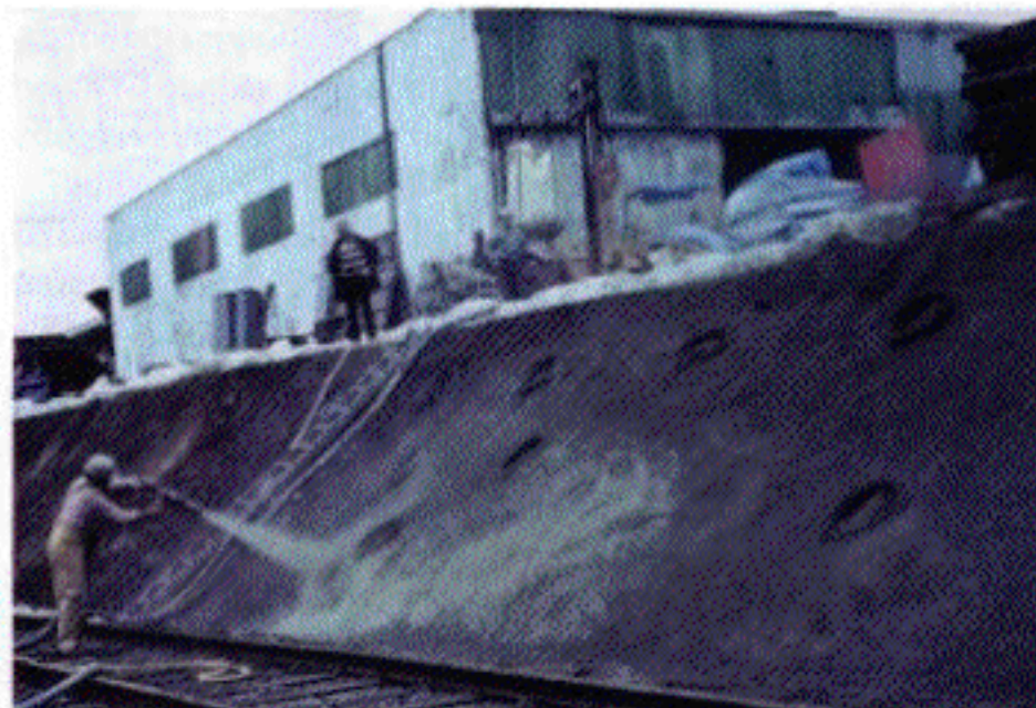
Figure 2. Railway embankment stabilization with SFRS, Burnaby, British Columbia, 1977.
