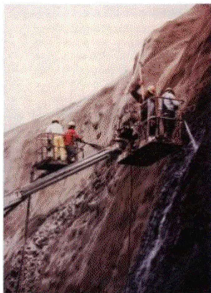
Figure 2. Shotcrete applied for slope stabilization.
