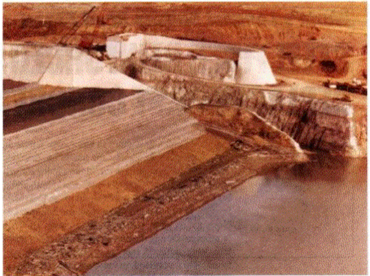
Figure 3. Initial stages of the sediment retention structure.
