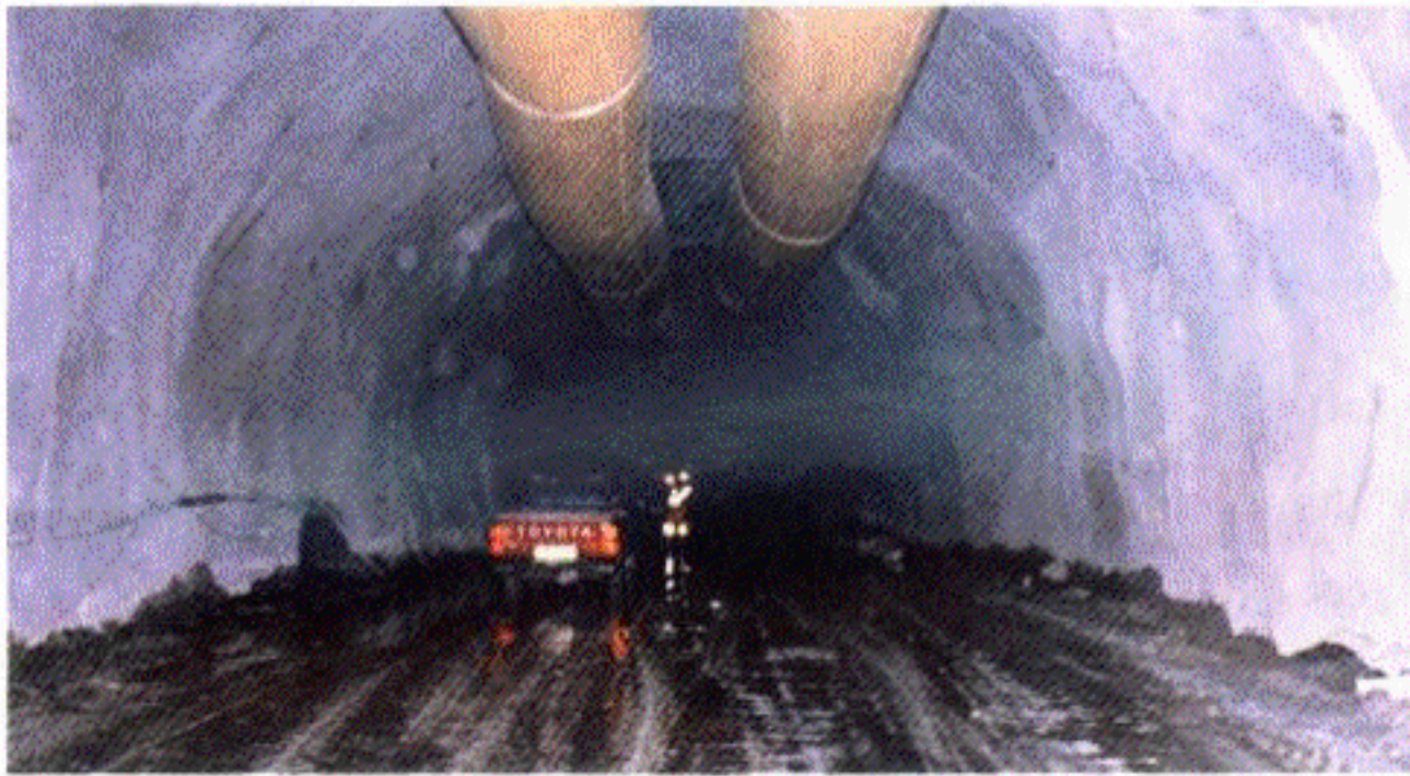
Figure 3. The final lining
