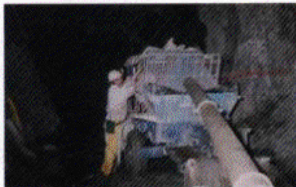
Photo 4. Pump receiving hopper and delivery pipe.
