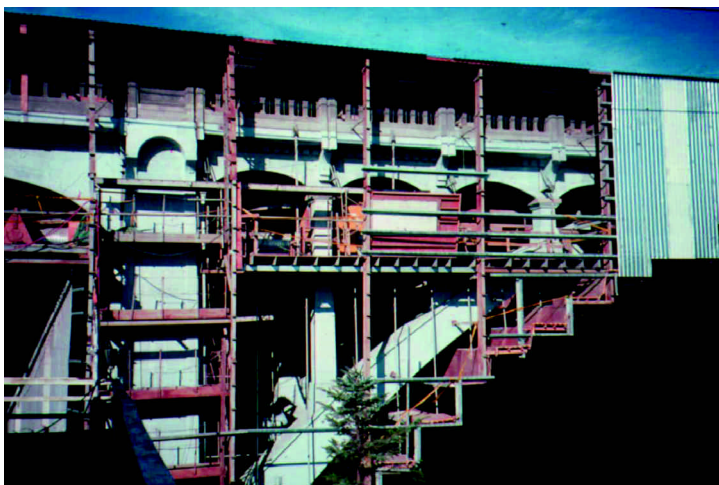
Figure 3. Repair of a highway bridge with dry-mix shotcrete.
