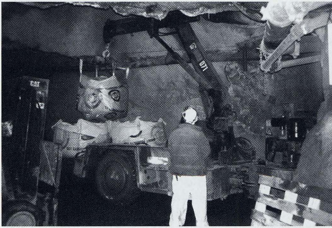
Figure 3. Small crane truck used to move bulk bags underground.
