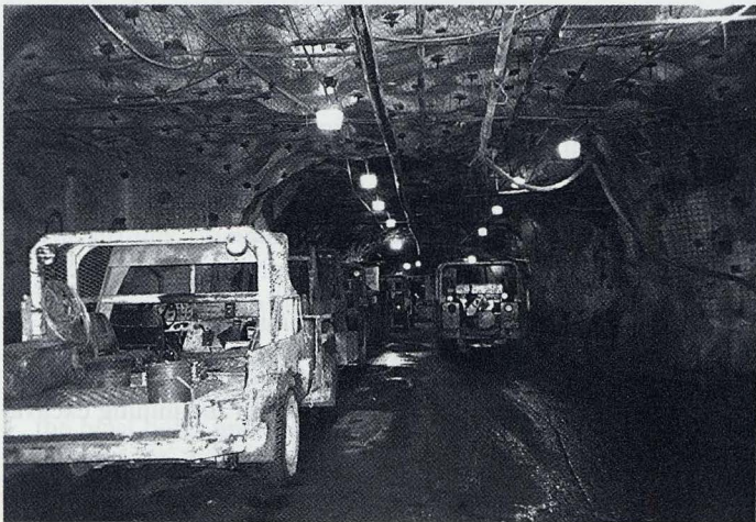
Figure 7. Rock bolts and mesh over shotcrete at a mine in New Brunswick, Canada.
