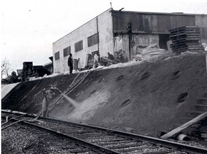
Figure 1. Stabilization of a sloughing railway embankment.
