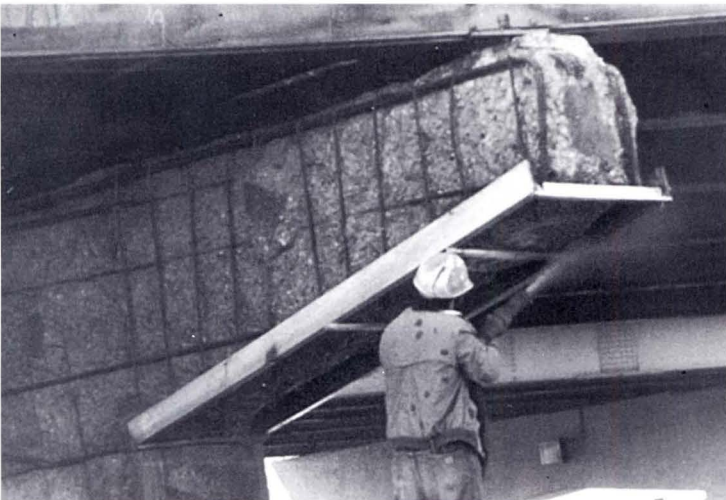
Figure 6. Restoration of hammerhead pier to original lines.
