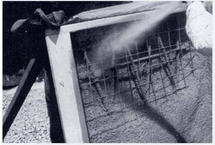
Figure 9. Shooting of preconstruction panel for cooling tower shell repair.
