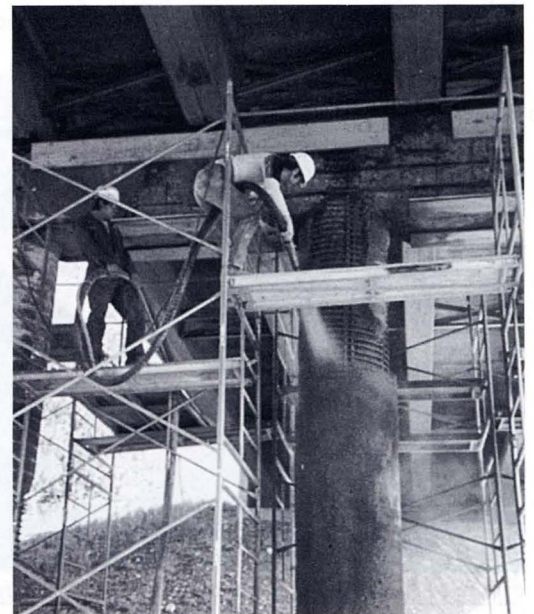
Figure 4. Repair of circular bridge pier.
