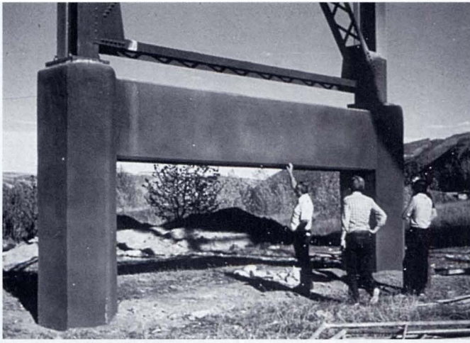
Figure 8. Completed bent.
