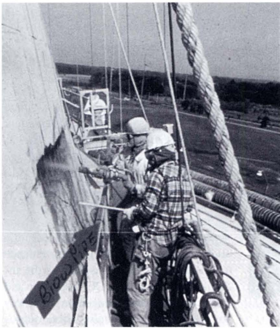
Figure 3. Use of blowpipe to remove rebound for cooling tower shell repair.
