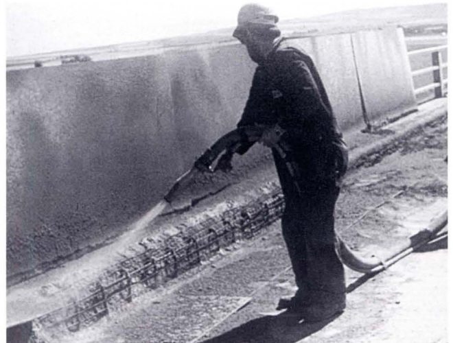
Figure 7. Shotcreting provides an efficient means of rebuilding bridge curbing.
