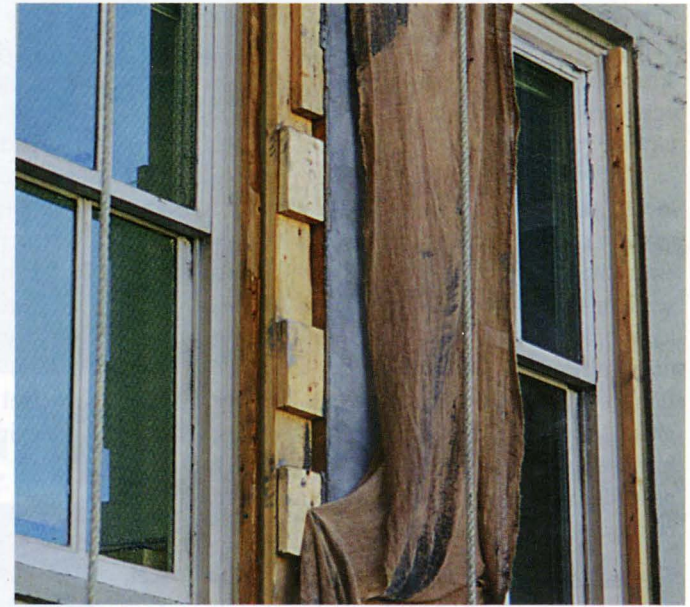
Figure 7: A look at the moist curing of shotcrete
