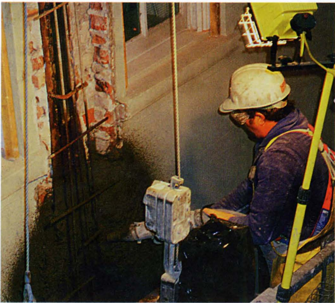
Figure 6: Close-up view of shotcrete application on column line.
