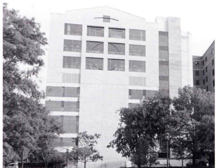
Seismic shear walls incorporated to add lateral support to an existing structure were critical to allow the addition of the top three floors in the vertical expansion of this medical center building
