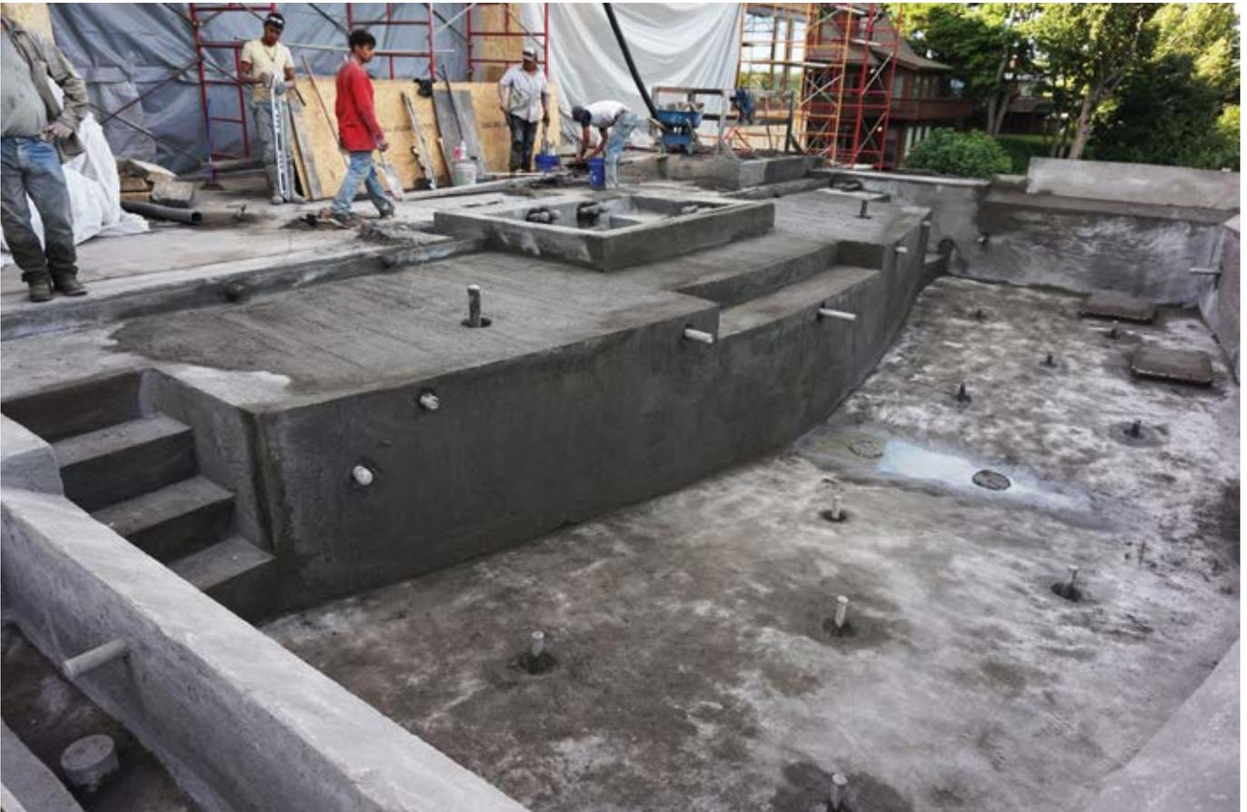
*Fig. 2: The finished shell shortly after being shot*
