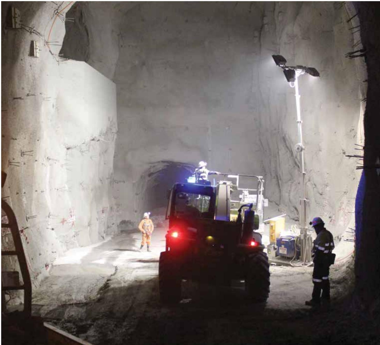
Fig. 4: Shotcreted transfer chamber
