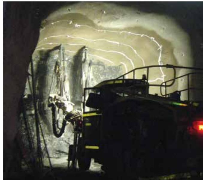
Fig. 2: Jumbo drill rig installing rockbolts through shotcrete
