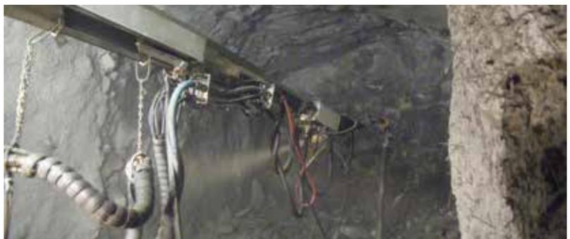
Fig. 6: Shotcreting in progress in undercut drill drive
